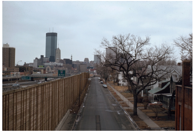
Wall barriers can help reduce roadway noise for residential areas adjacent to freeways.
