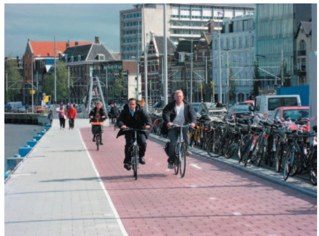
People will use different modes within one trip, depending on where they are traveling.
