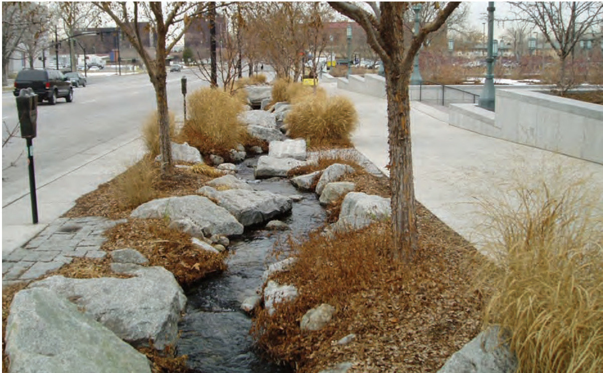
Stormwater retention elements such as this treat water on site and provide a pedestrian amenity.
