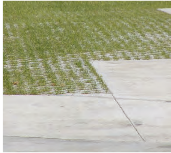
Permeable paving reduces runoff and filters stormwater.
